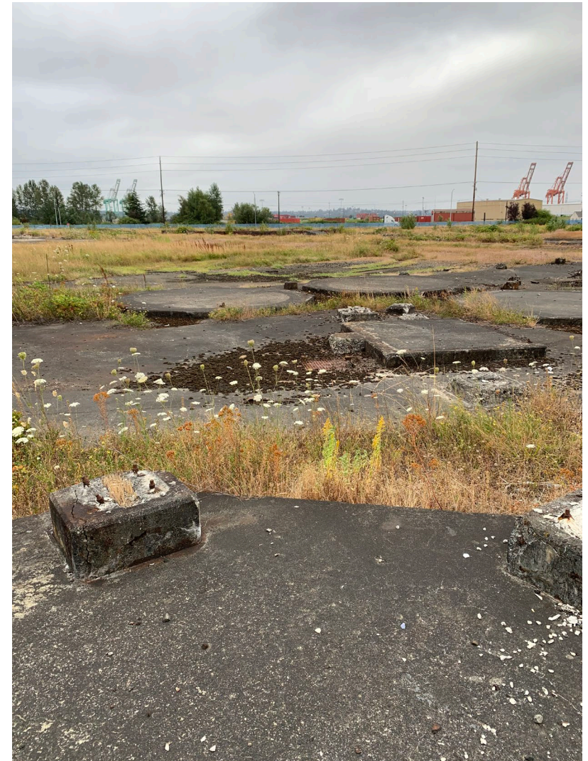
First Person View of Foundations
